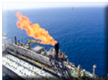
Live Offshore and Onshore Flare Inspections
