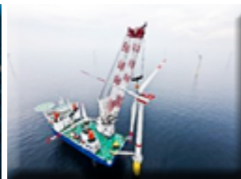
Offshore cranes - Lifting Over Watch
