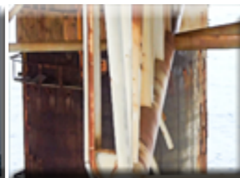
Under Deck and Splash Zone
