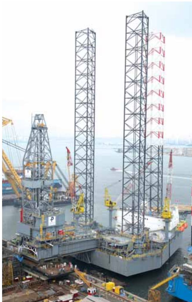
The KFELS Super B Class rig is equipped with cantilever skid-off capabilities.
