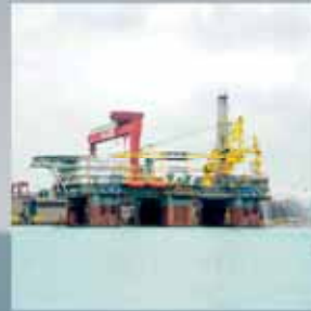
11 PV Drilling V
