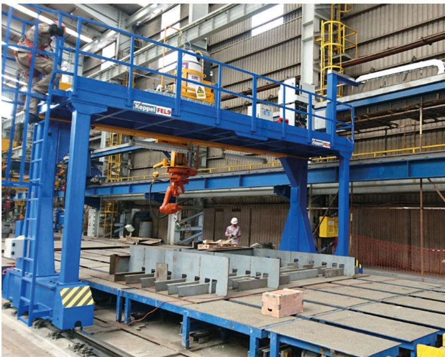
Keppel FELS installed a gantry-mounted robotic welding system on the panel production line, which has improved accuracy of welding and reduced man-hours.
